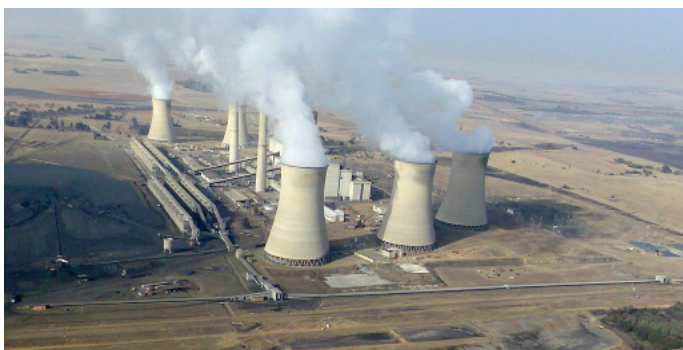
Arnot coal plant, South Africa. Photo: Gerhard Roux
